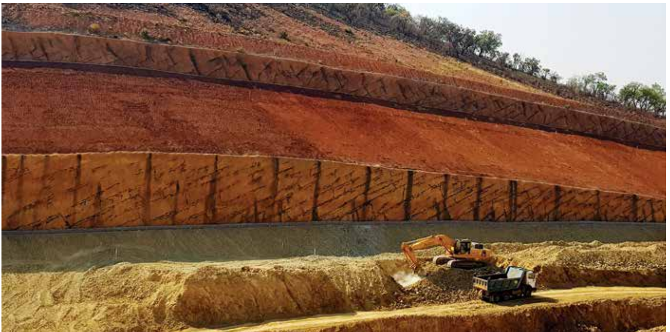
Fig. 4: Completed works on the eastern side
