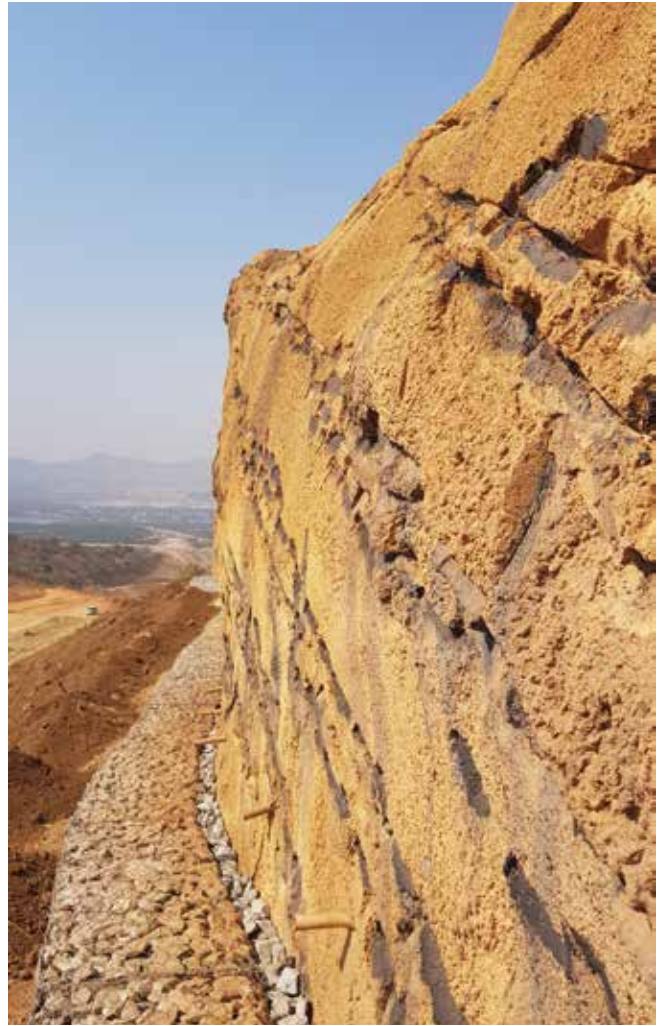
Fig. 3: Completed wall with aesthetically pleasing outcrop and shadowing
