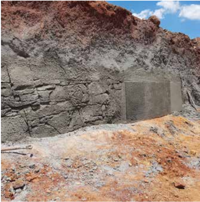
Fig. 2: Sample of rockscaping, woodfloat, and brushed finish for the clients to inspect
