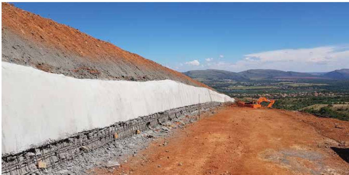
Fig. 1: Shotcrete finish—woodfloated and brushed
