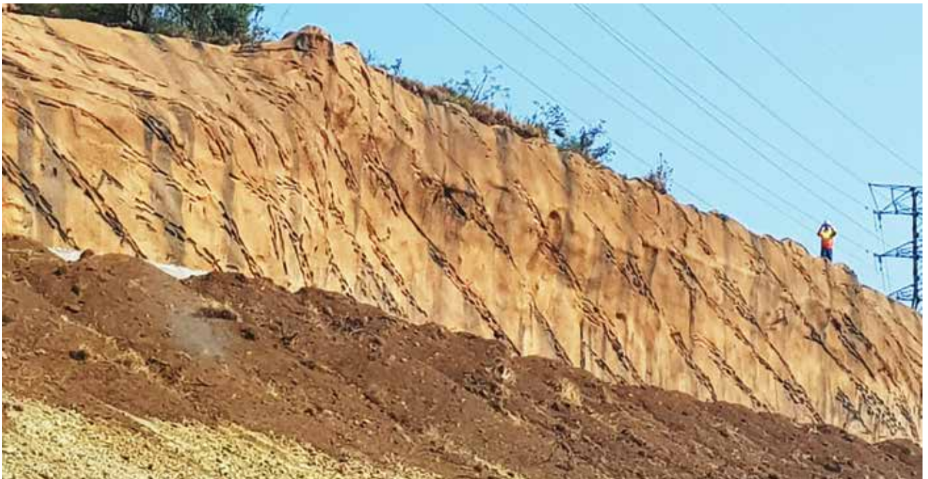
Fig. 5: From an absolutely flat-topped and flat-faced piled wall to this
