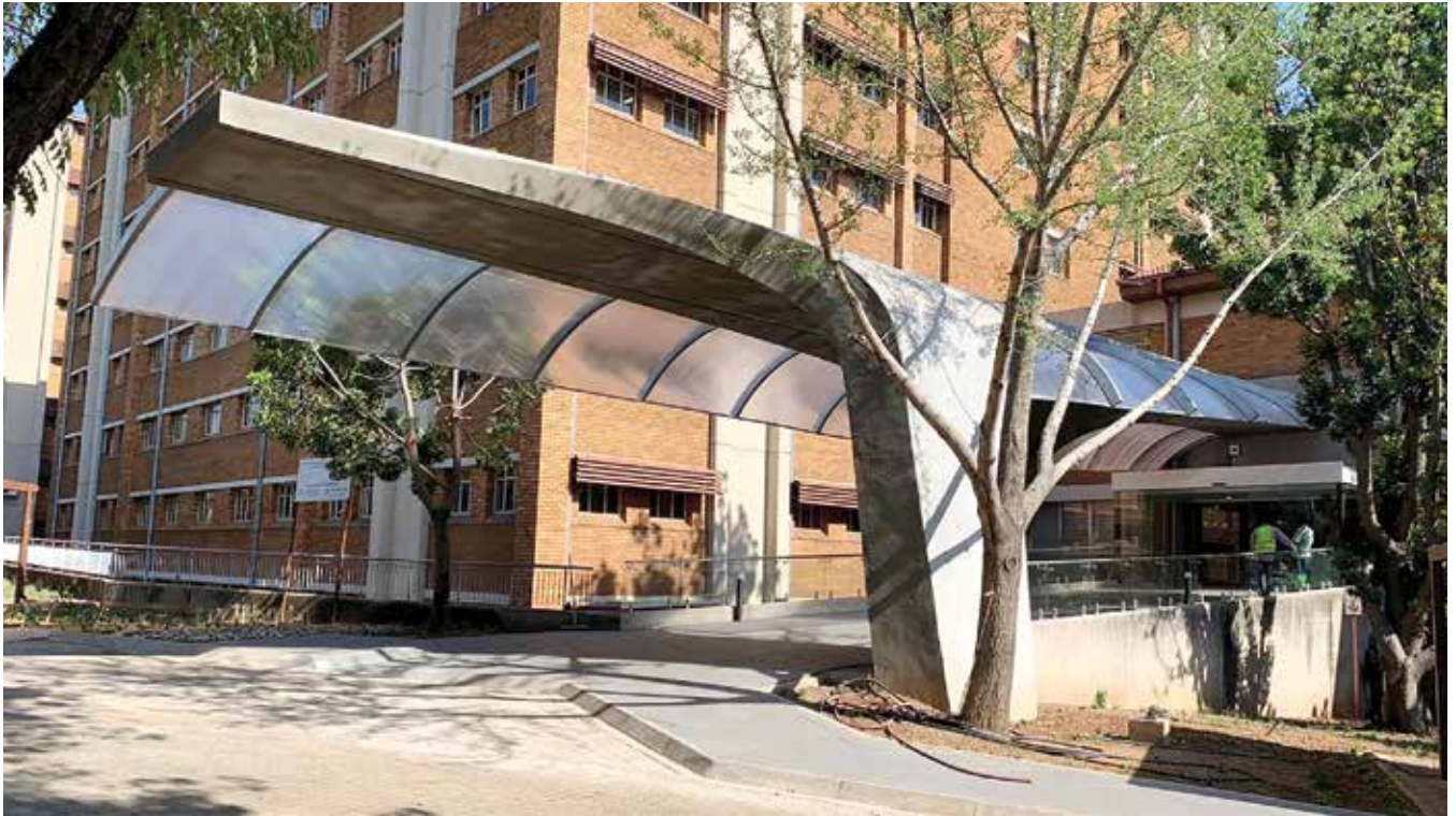
Fig. 6: A side view of the finished structure before painting
