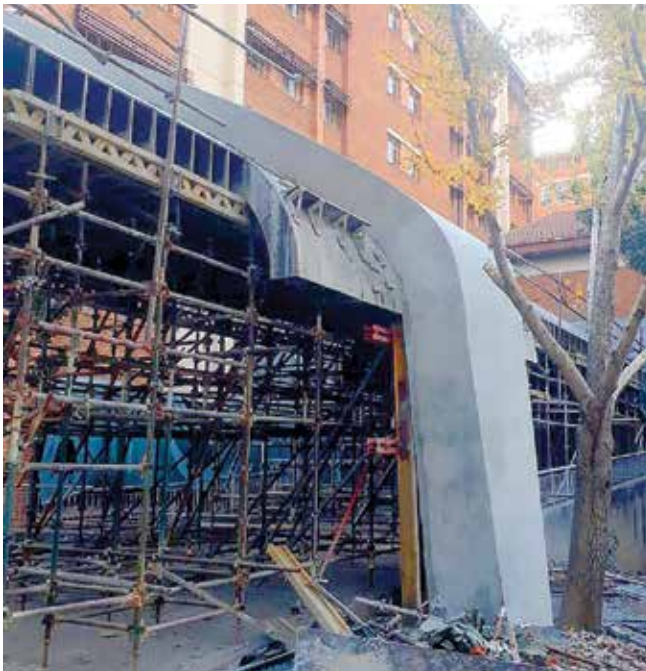
Fig. 5: A view of the curved column with canopy sitting on the form
