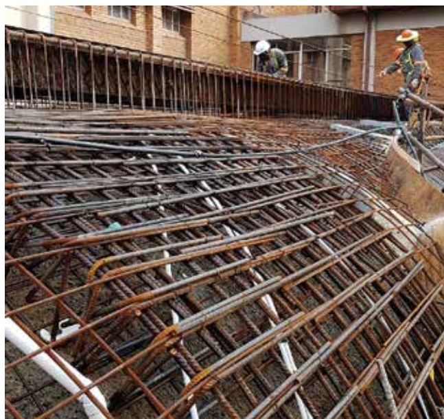
Fig. 3: Complex reinforcing steel for the canopy
